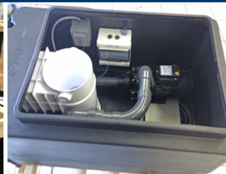
Inside the Excellence Compact filtration unit
