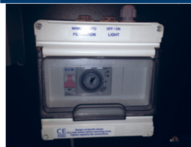
Control box and pump protection with clock
