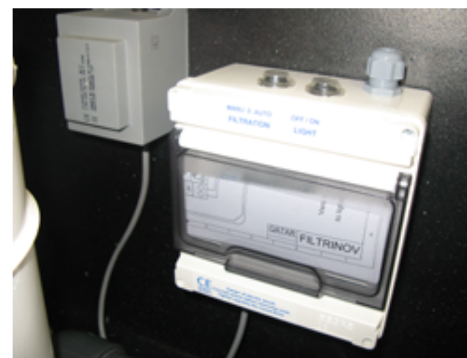
12V 100VA transformer for 1/2 LED
